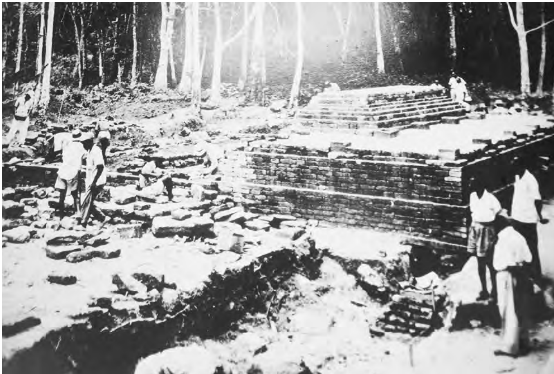
Fig. 4 Excavation and restoration of a Hindu temple platform, Chandi Bukit Batu Pahat, Merbok, Bujang valley, Kedah, Malaysia. This riverine site, with access to the estuary of the Merbok River, was one of the early centres for intermediate trading on the West Asia–China route (Photograph courtesy of the Museums Department, Malaysia).
