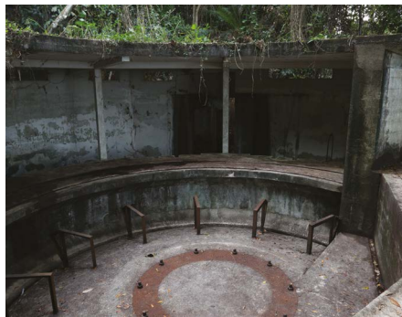
FIG. 3: GUN FLOOR CONSISTING OF OVERHEAD CONCRETE CANOPY, GUNNER'S PLATFORM, AND HOLDFAST BOLTS FOR A TWIN 6-POUNDER GUN. (CREDIT: YOUNG WEI PING)
