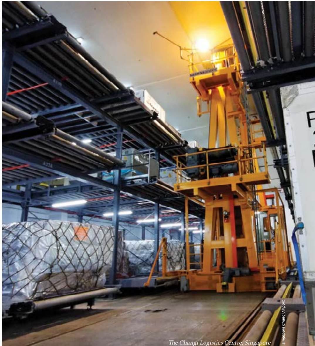
The Changi Logistics Centre, Singapore
