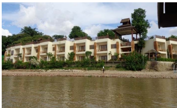
Construction of hotel inside Archaeological Zone along river
