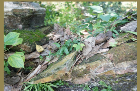
REMAINING FLAT TERRACOTTA TILE PROTECTING THE GABLE. (CREDIT: HÉLÈNE NJOTO)
