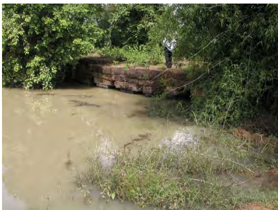
Figure 4 Laterite bridges identified along the royal road from Angkor to Phimai
