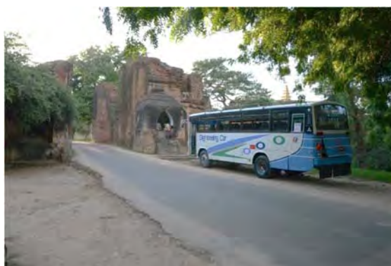
Traditional pulling up to nats at Tharba Gate threatens stability
